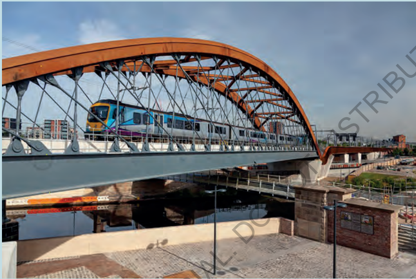
Figure 2.1 The asymmetrical network arch bridge over the River Irwell, Ordsall, Salford
