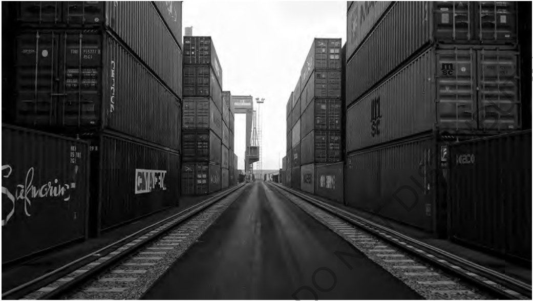
Figure 7.6 ASC rail tracks on gravel beds (by kind permission of DPW Antwerp Container Terminal and photographer Frank Bahmuller)
