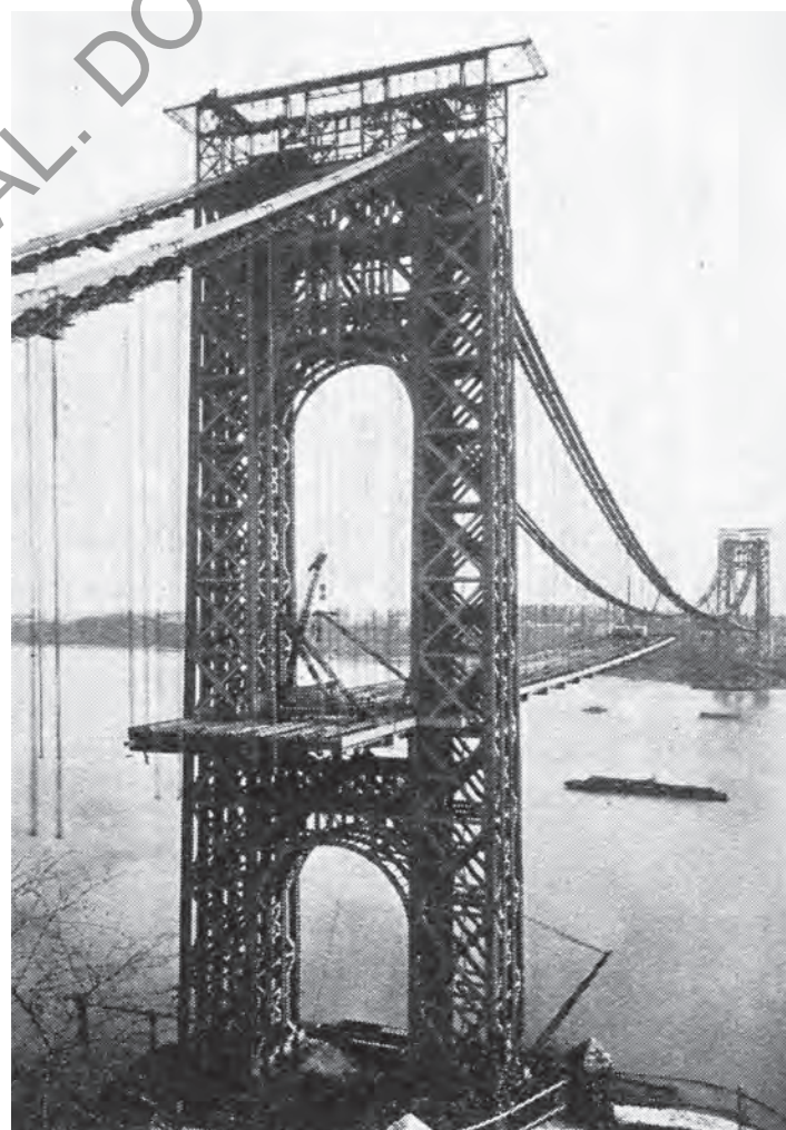
Figure 1.14 George Washington Bridge, New York
