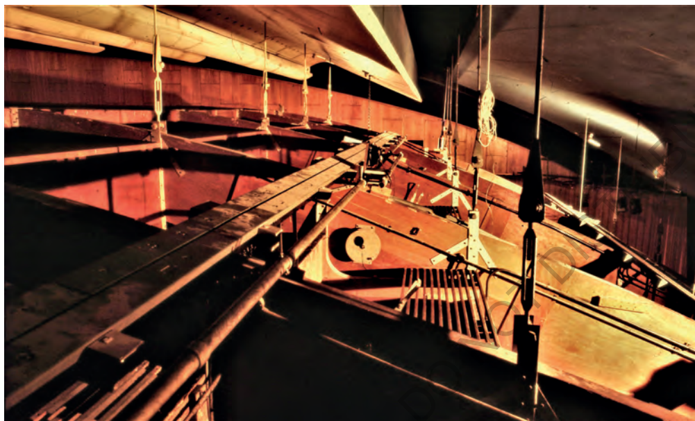
Figure 18.1.4 Canopy suspension
