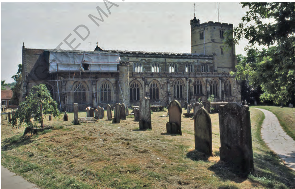
Figure 19.1.1 View of the church from the north-east, showing the temporary cover
