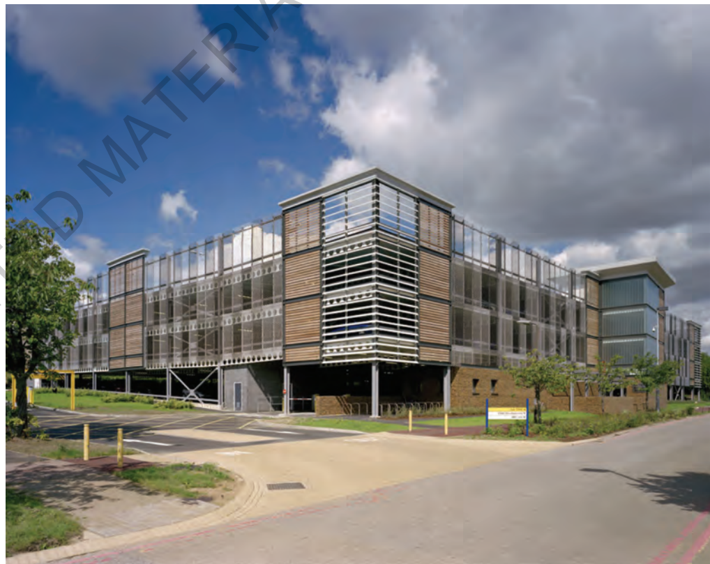
Figure 2.2 Typical steel-framed car park (courtesy of Milton Keynes University Hospital NHS Foundation Trust)
